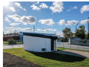
The BOD in Copenhagen is said to be Europe's first 3D printed building.
