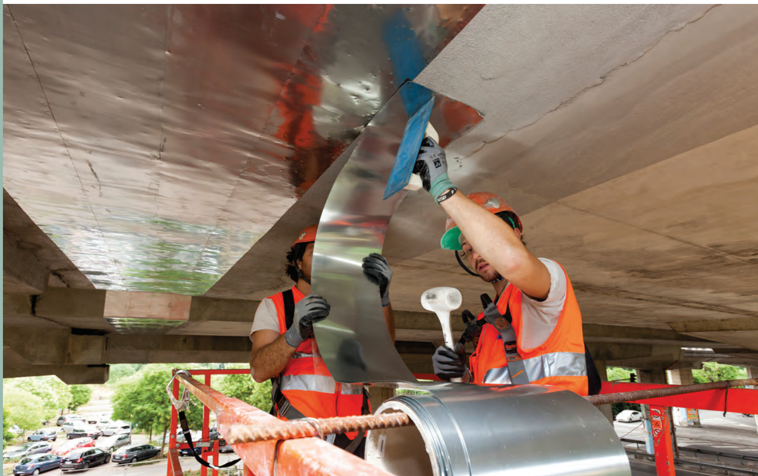
BELOW: Applying Mapeshield E 25 directly on the external surface of concrete.
