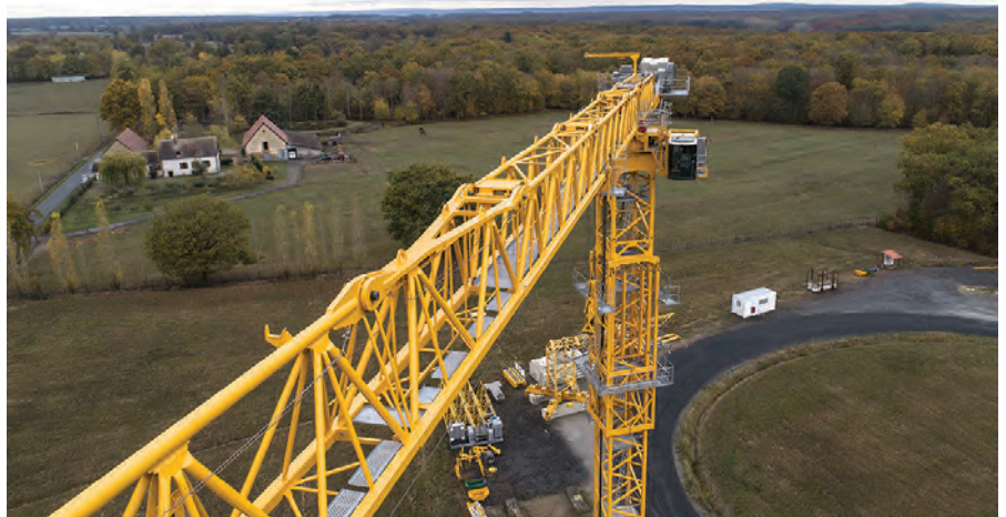
ABOVE: Potain MDT 809, the largest topless crane ever built by Manitowoc.
