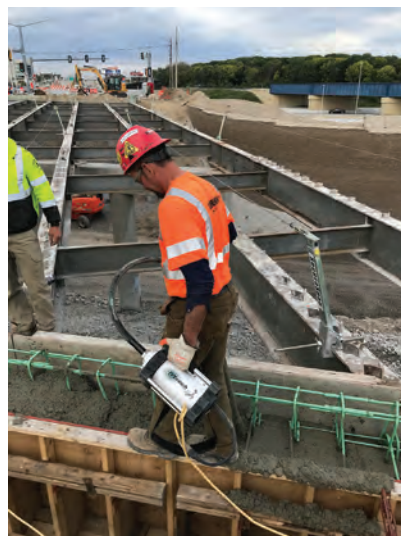
ABOVE: Minnich Auto Vibe vibrator monitoring systems.
