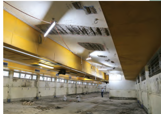
TOP AND ABOVE: Mapeshield I was used to repair concrete at the Sha Tin racecourse in Hong Kong.
