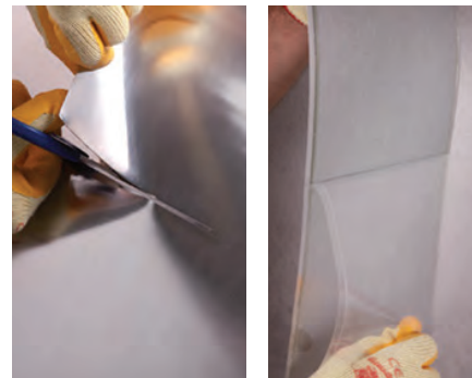
The Mapeshield E 25 self-adhesive zinc plates can be applied directly on the external surface of concrete.
